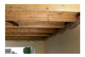
**2.** Remove the existing plasterboard ceiling to expose the timber joists
