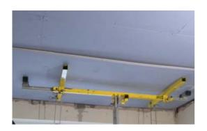
**10.** Install the second layer of 15mm acoustic plasterboard (with FlexiSound attached). Lift the board up to the ceiling and fix in position using the 50mm self-drilling screws, sandwiching the FlexiSound between the two plasterboards. Stagger the joins by starting at the opposite side from where you started on the first layer. Remember to leave a 5mm gap around the perimeter. A screw should be used every 200mm on each furring channel.
