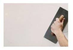
**12.** The ReductoClip Ceiling System is then ready for standard plasterboard finishing. A plaster skim finish is most common but heavy duty backing paper can also be used.
