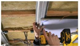
**8.** While holding the acoustic plasterboard in position use the 25mm self-drilling screws to secure the board into each ReductoClip furring channel. Screw the fixing in place until the screw head is flush with the plasterboard. A screw should be used every 200mm on each furring channel. Once the first plasterboard is in position, apply the next board butting up tightly to the previous board and continue.
