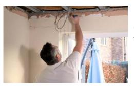
**6.** Before installing the first plasterboard layer, mark the locations of the furring channels on the surrounding walls in chalk or pencil. This will help you to locate the position of the furring channels later once the first layer of plasterboard is on and furring channels are no longer visible.
